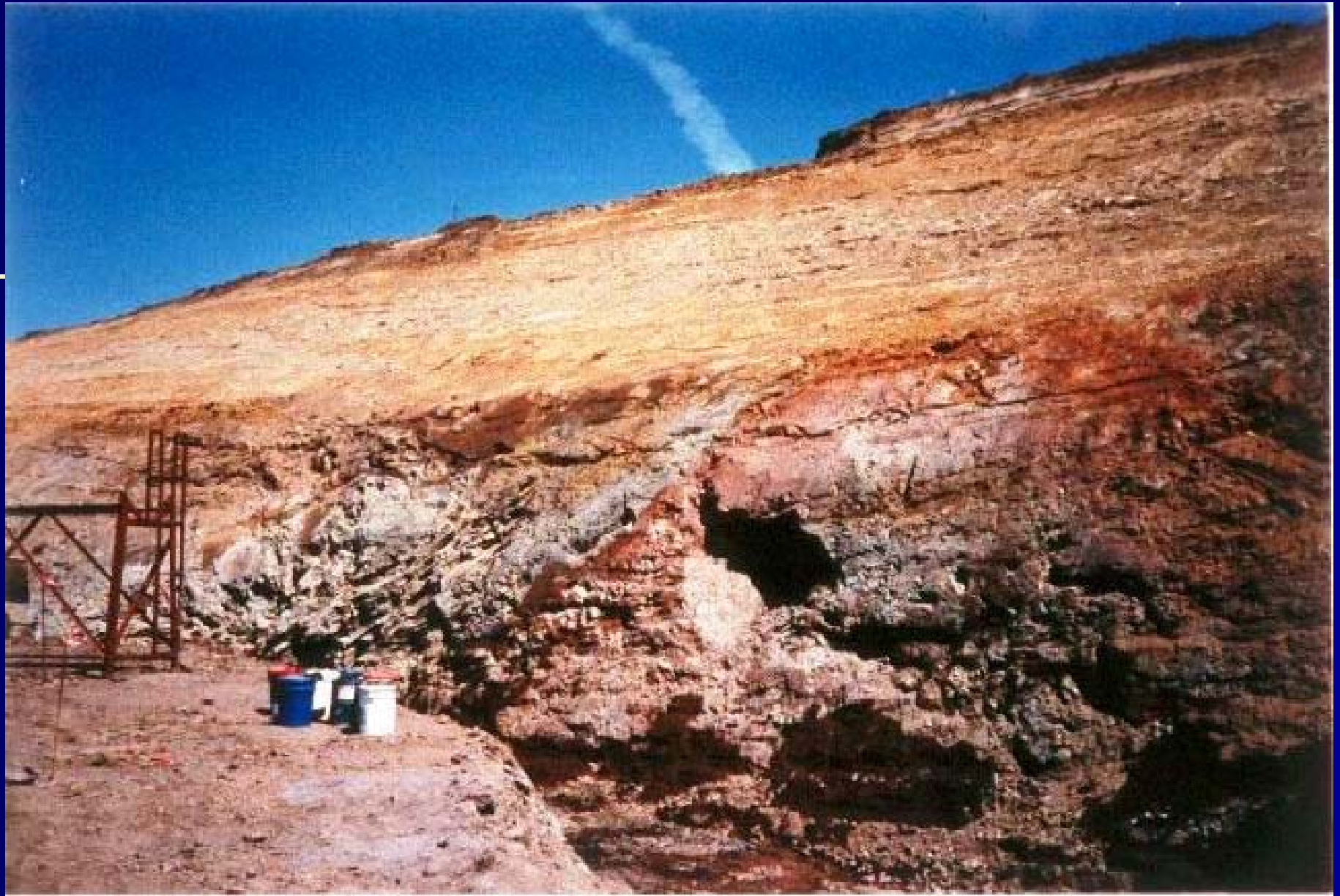
Right abutment area on June 30, 1987. Dark material at top is the "slimes", lighter material beneath is the impervious borrow, and the lower dark zone is the flow breccia.
