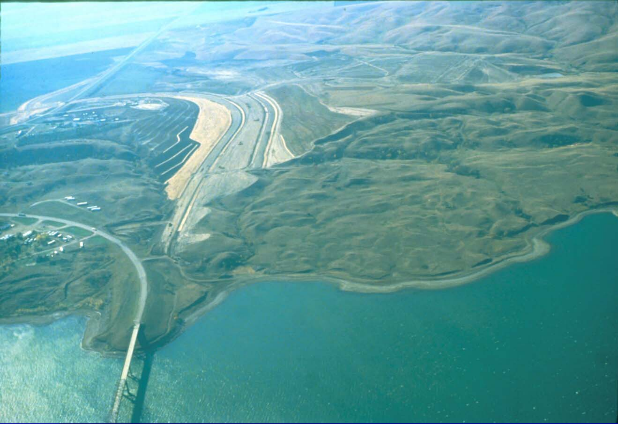
Excavation of slide near its head. (Slide courtesy of Vern Schaefer)
