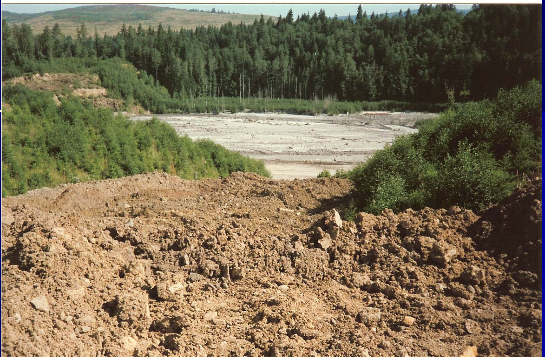
Unstable stockpile slope of old glacial drift gravels excavated from the left abutment area of the Mt. St. Helens Sediment Retention Structure.
